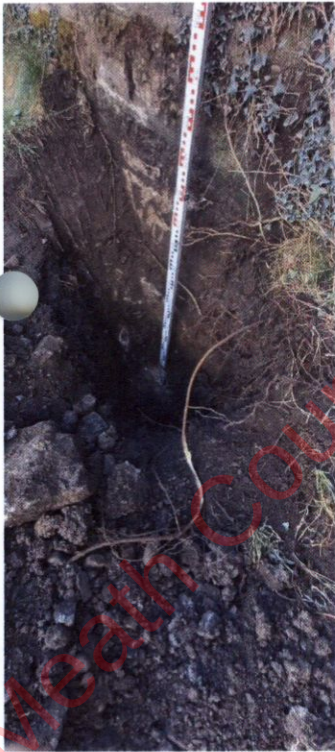
Beaumont Bridge (Trial Hole 8)
