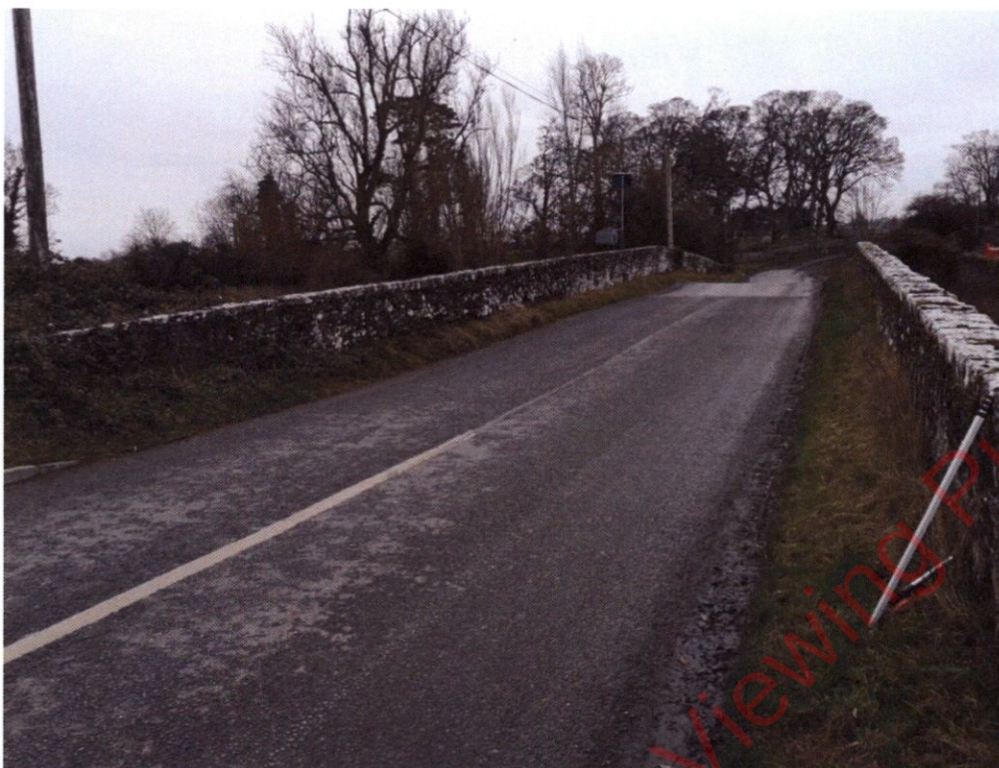
Photograph B-1 – Bridge surface looking south
