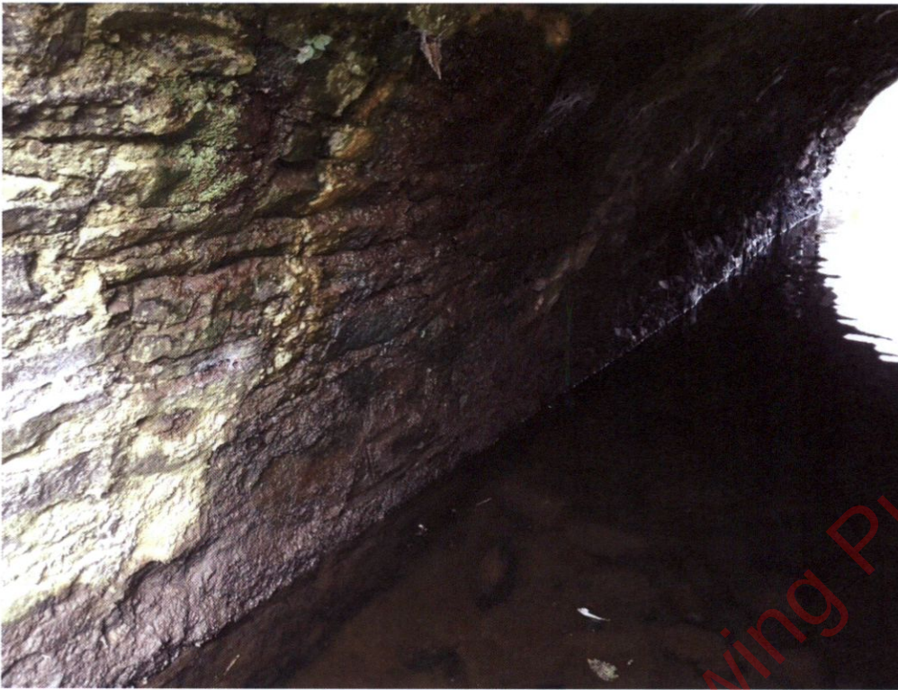
Photograph B-21 – South face of pier 5
