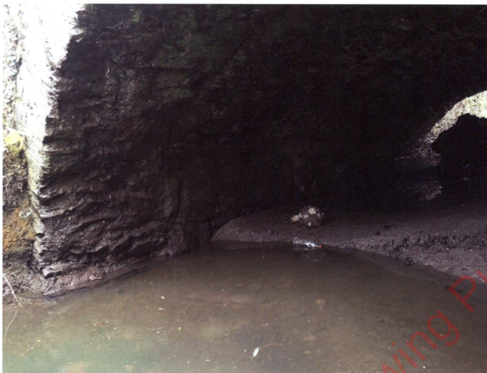
Photograph B-13 – South abutment
